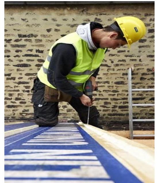
Insulated custom roof panels and hinged roofs
